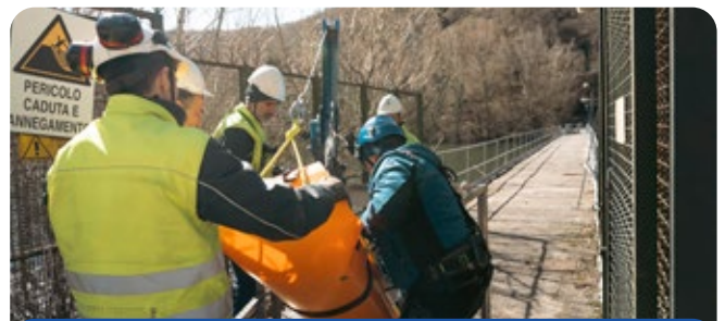
Confined space dam
