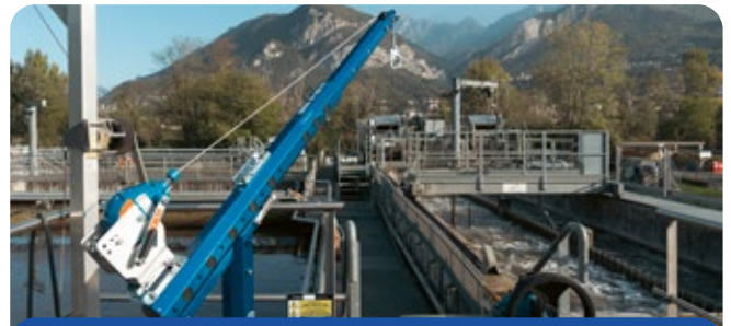
Confined space tank
